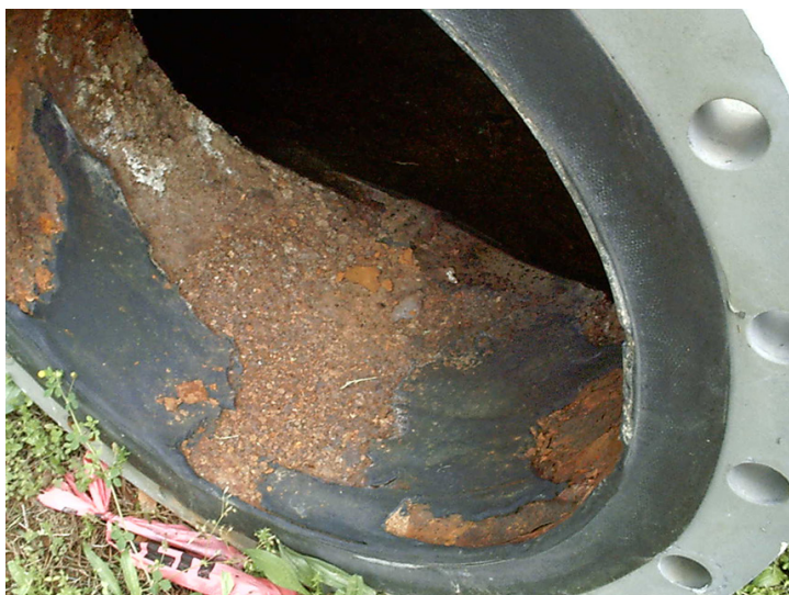
Chemical attack behind a rubber lined carbon steel pipe
